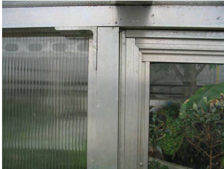
Figure 3. Close-up of the 1inch (2 cm) aluminum angle pieces holding the 1.5 x 1.5 inch (3.8 x 3.8 cm) aluminum tubing and storm door.
